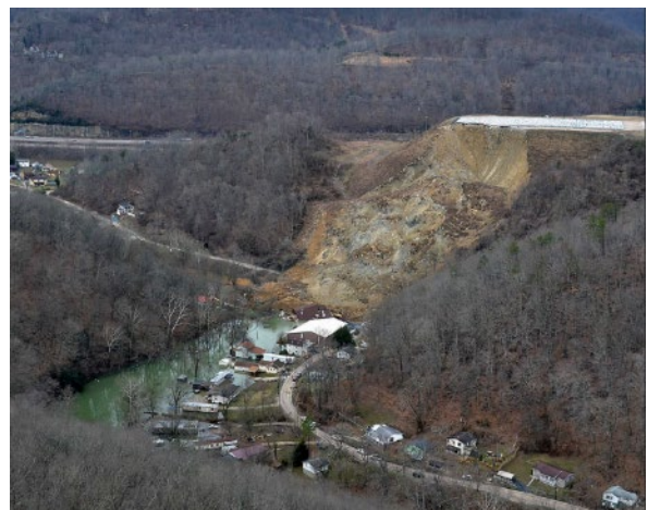
Figure 5.7-1. Yeager Airport Landslide of 2015
